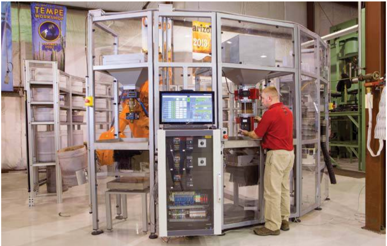
The control console has a large monitor and holds several EI controllers. Bryan Chevrie demonstrates how easy it is to install a MagnaValve.
