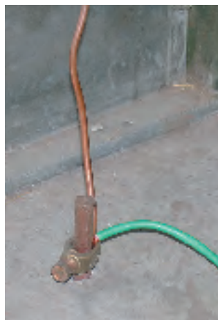
Ground to earth
