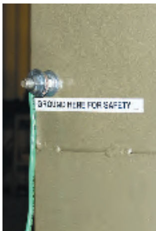
Ground from cabinet
