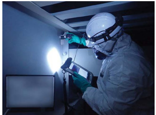
Fig. 5 UV-CC at a steel bridge repair work site.
