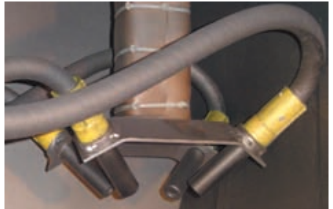
Pressure blast nozzles (auto touch-up)
