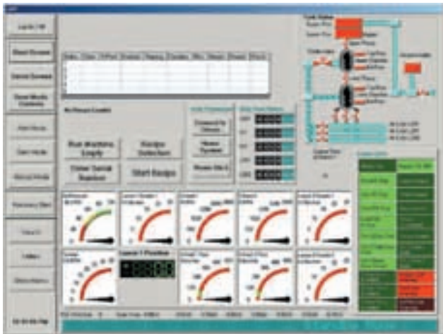
Operator interface with real-time monitoring in an electric control system
